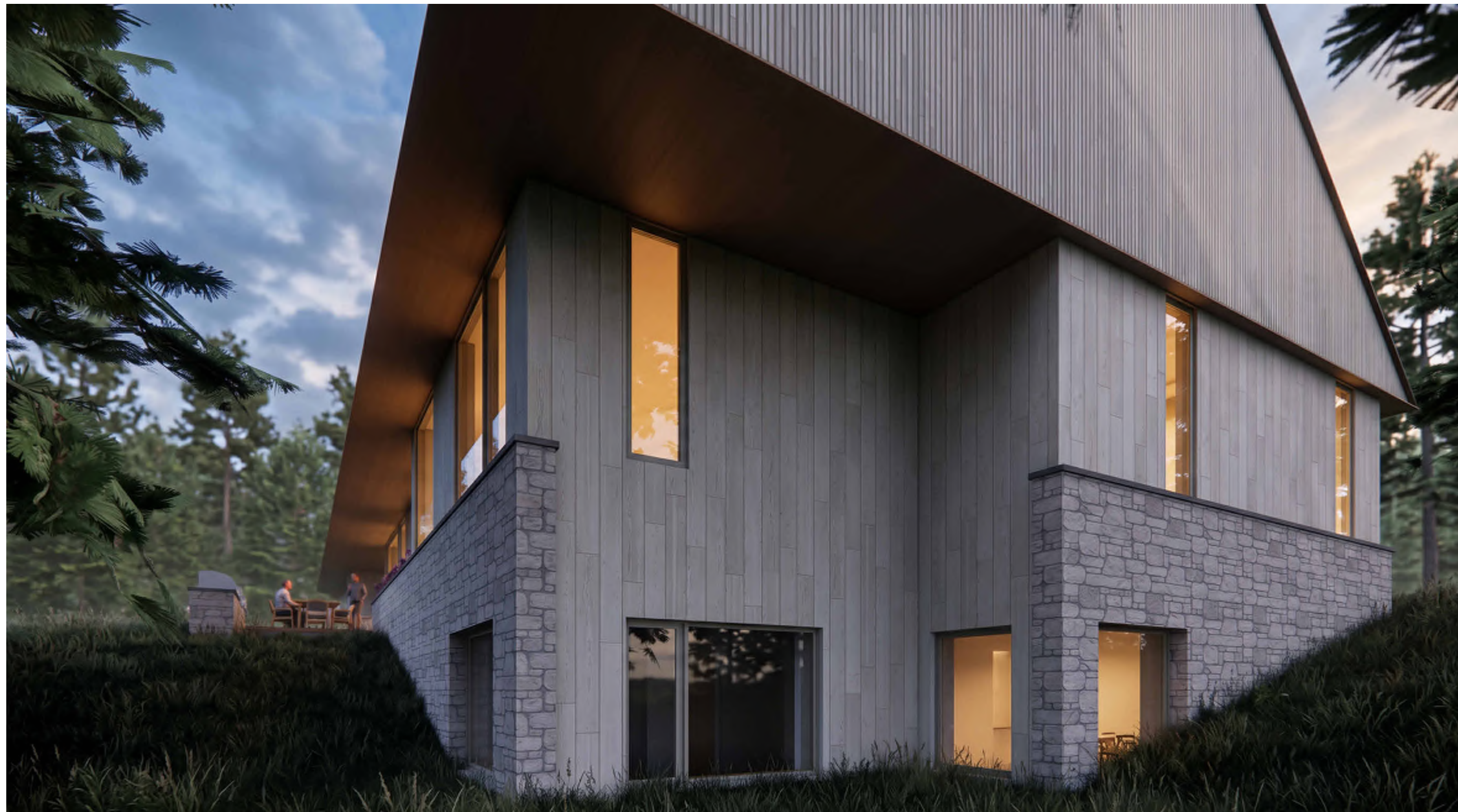
NORTHEAST CORNER DOUBLE HEIGHT SPACE MATERIALS
